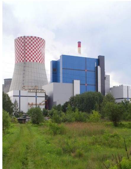
The Lagisza Power Plant in Poland features a 460 MWe Amec Foster Wheeler supercritical, vertical-tube CFB boiler.
